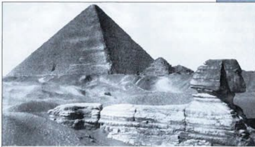
Photograph of 1921 clearly showing the crack separating the main part of the Sphinx from its rump. This was due to a structural weakness caused by the burial of a later Pharaoh (possibly 26th Dynasty) beneath the Sphinx. This crack was filled with cement in 1926 by the archaeologist Émile Baraize. Photo: Collection of Robert Temple
