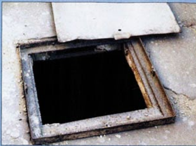
Modern cover to the entrance of an underground chamber in front of the Sphinx. The tunnel leading off beneath was blocked by Henry Salt in 1817.
